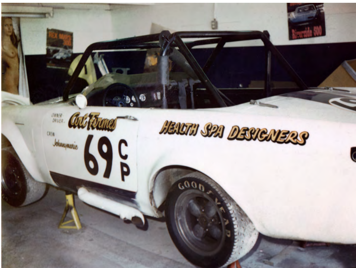
The Guldstrand Tiger during re-painting and re-lettering at the Guldstrand Engineering shop. Note the over spray in the wheel wells and on the tires. Steve Feinberg painted the lettering and applied the gold leaf. The fabricated dash with the ignition control is visible. Photo: Dick Guldstrand, 1974.
